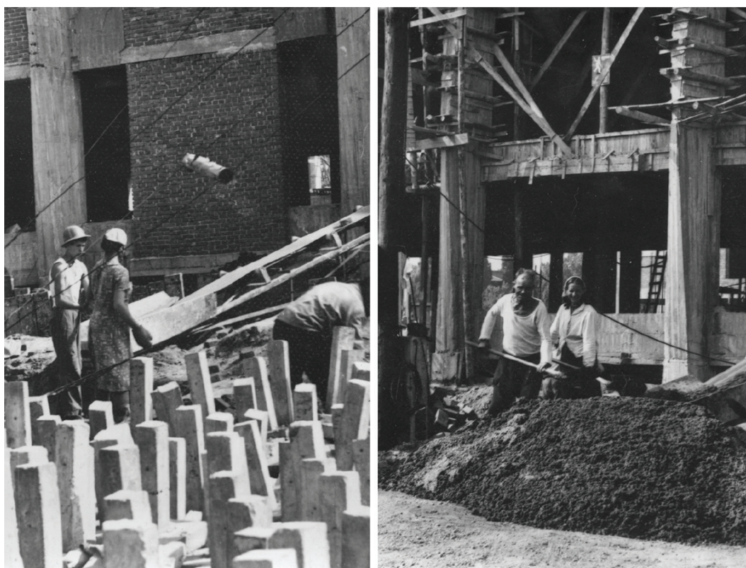
Figures 1 and 2. On the construction site of the Television Centre in Bucharest. ©TVR.
