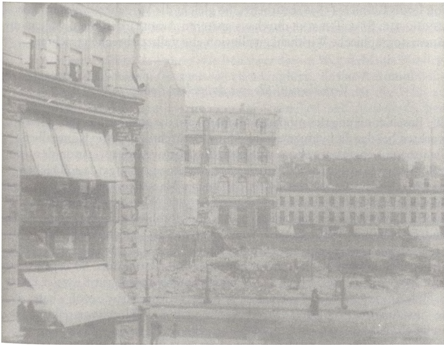
DEMOLISHING THE STAR THEATRE (American Mutoscope and Biograph 1901)
