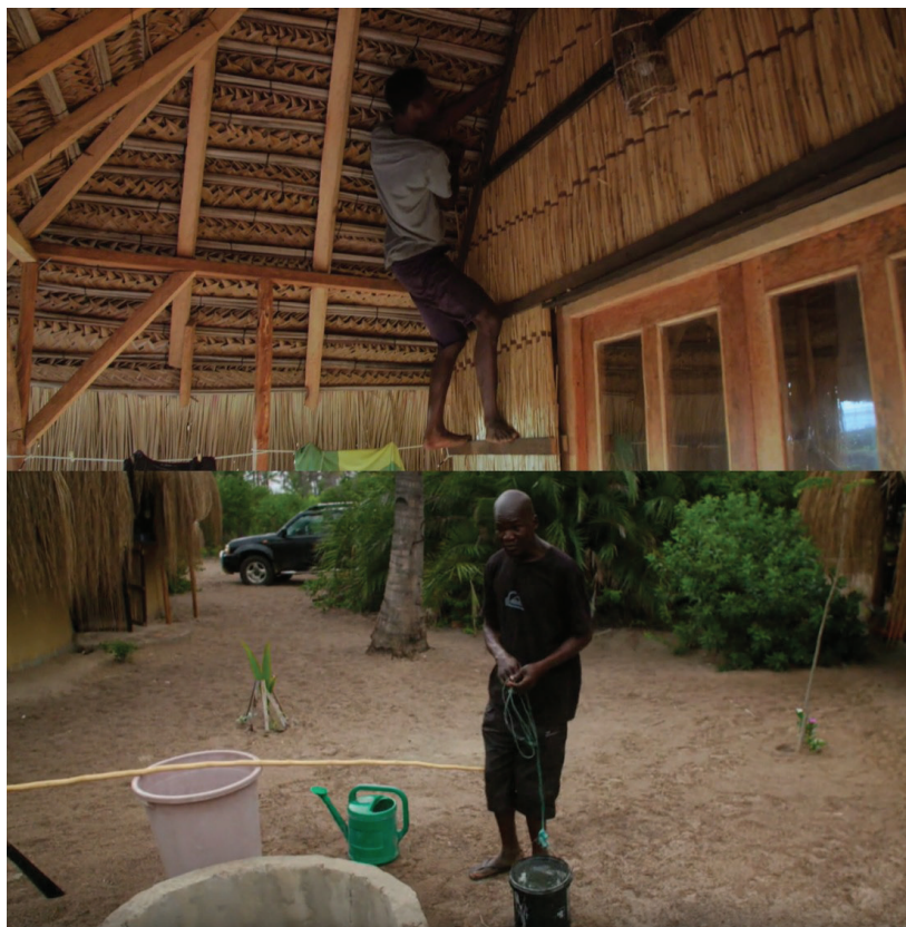
Figure 12. Local workers are called in to fix what the visitors break.
