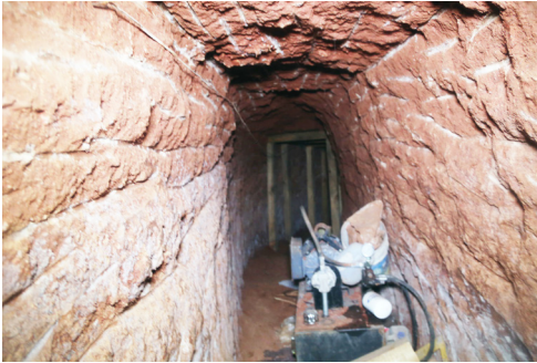
Figure 2. Tunnel found in Naco, Arizona, in 2015: dug through soil and clay. Source: U.S. Customs and Border Protection
