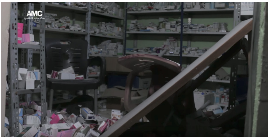
Fig. 3: AMC video published on YouTube documenting the damage to the interior of Al Rahmah hospital in Khan Sheikun.
