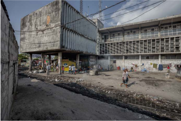
Fig. 5: Sammy Baloji, Site Cielux, Municipality of Masina, Kinshasa, 2013 (OCPT building).
