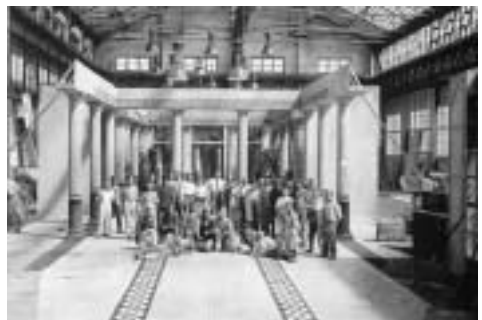
Fig. 2.9 – Interior of the JOFA-Atelier.
