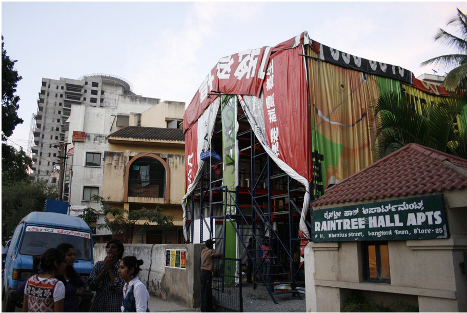
Figure 15: The Jaaga building made of pallet racks. Image source: Wikipedia.
