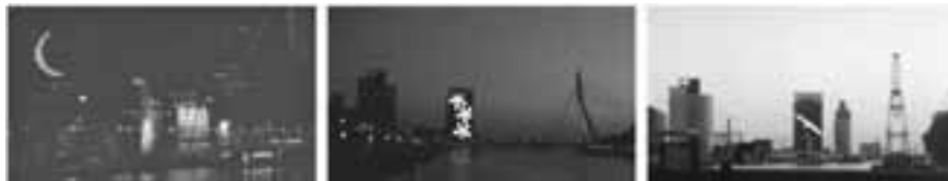
Fig. 11: The KPN building as it changes throughout the day.
