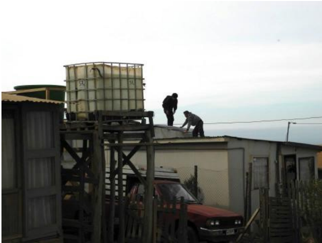
Fig. 27. Antenna installation on Mariposa Hill.
