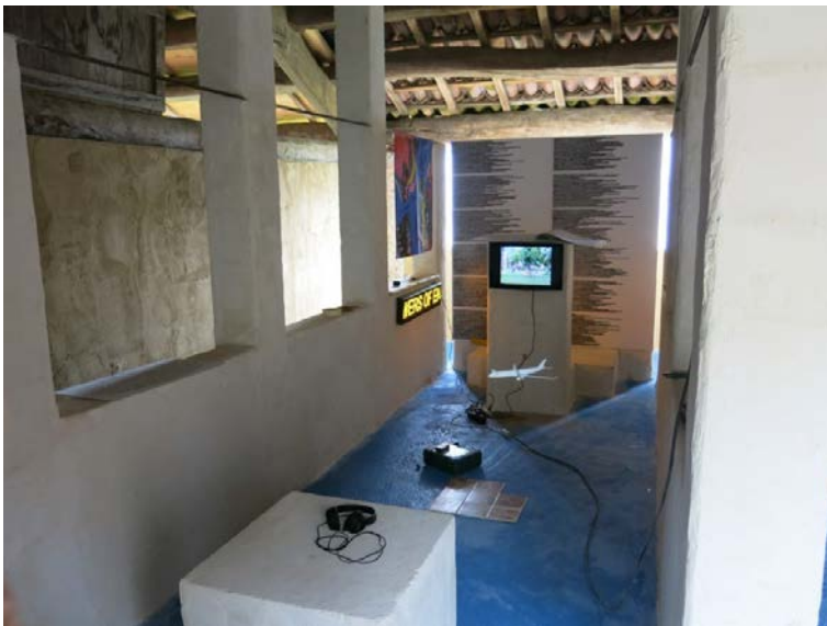
Fig. 5: Alberto Frigo's renovated barn in the Italian alps, under construction now to showcase his project.
